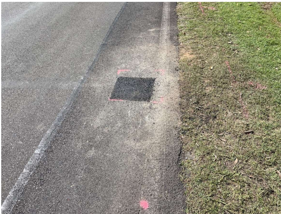
Photo 4 - Completion of Backfill (CBR A)
